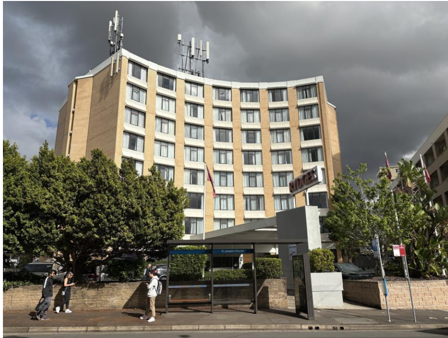
Figure 1: 3-19 Missenden Road, Camperdown, viewed from the north-east
